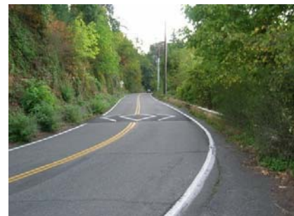
Uphill shoulder needed on a portion of lower Montgomery
