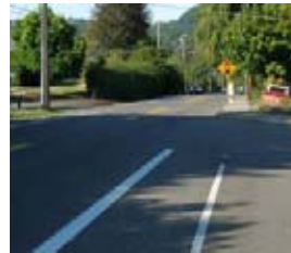
NB bike lane drops approaching Vermont
