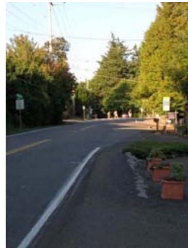
Location of uphill shoulder/bike lane on Patton
